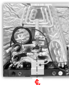
Figure 12.4 VERTICAL/UPFLOW CONFIGURATION (Uncased/Cased Coil)
