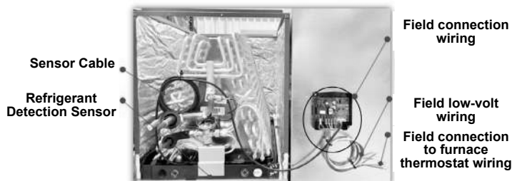
FIGURE 12.3A - MITIGATION CONTROL SYSTEM
